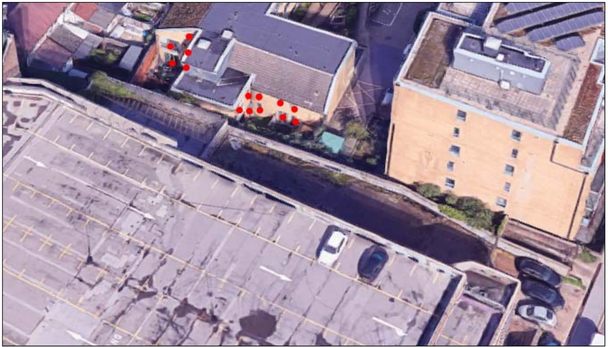
Figure 26 – Location of impacted windows within block to the rear of 53 Whytecliffe Road South.
